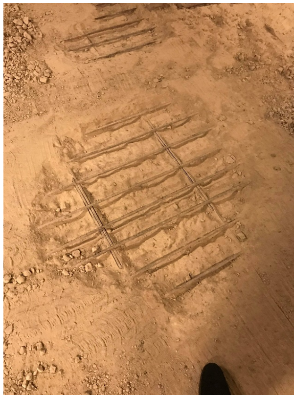
Frisk armering, men skadet betong
