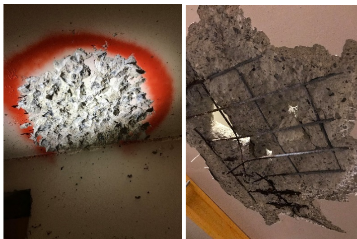
Steinreir i underkant dekke
