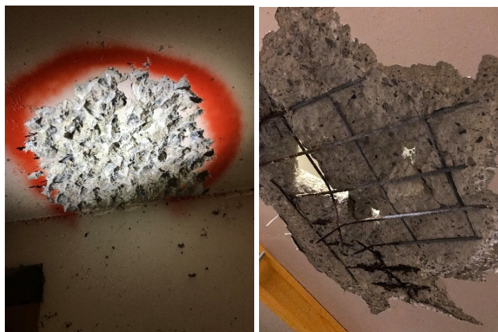
Steinreir i underkant dekke
