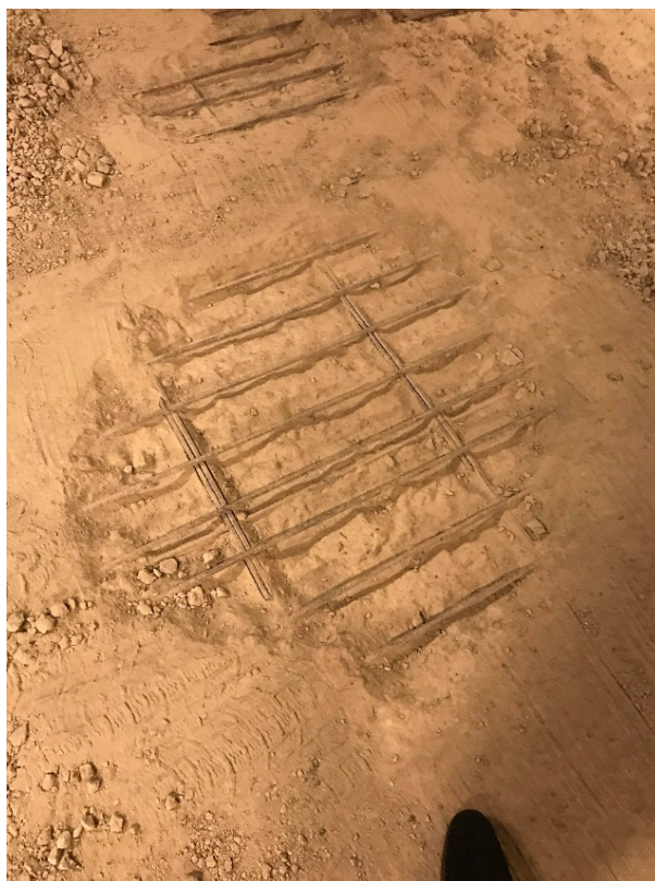
Frisk armering, men skadet betong
