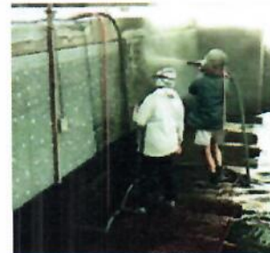
Fig 15. Spraying mortar
