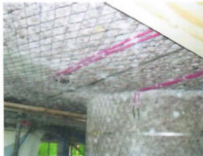
Fig 14. Titanium mesh [8]
